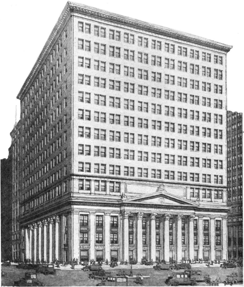
New Home of the Federal Reserve Bank of Chicago In Course of Construction
