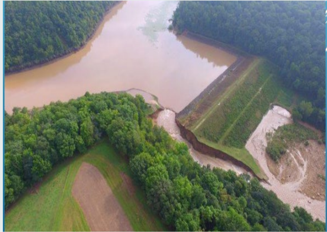
Breach of Seas Branch Dam, Vernon Co, WI, Aug 2018
