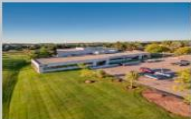
2 Changan US R&D Center
