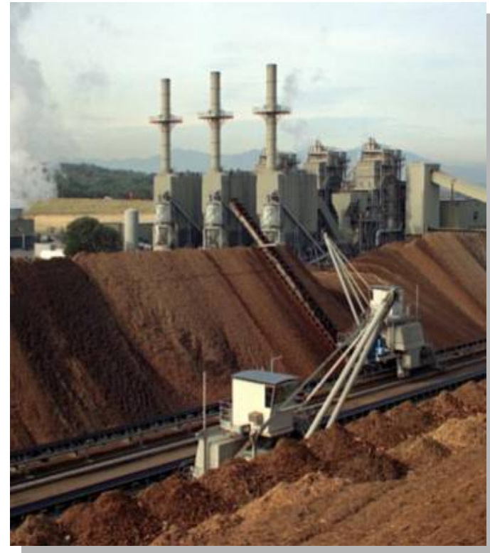
49-MW Wheelabrator Shasta plant, California
