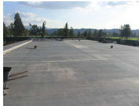
Manure Digester, Chino, CA
